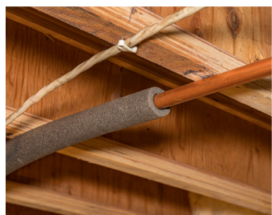
Improve pipe insulation to reduce the risk of a flood from burst pipes in winter.
